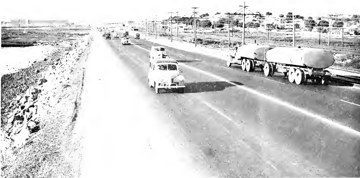
Richmond Access Road. Looking north from El Cerrito Overhead. Construction is across deep marsh. Trolley tracks on right were constructed by the Maritime Commission to serve ship yards. Southern Pacific main line is to the right of trolley tracks
